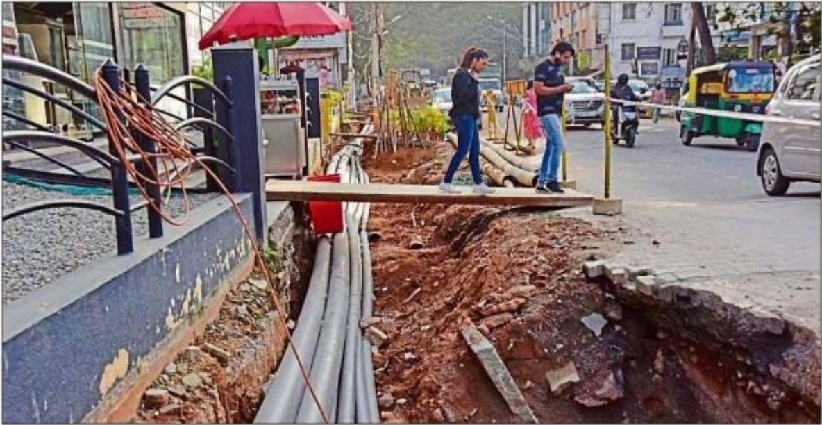
Footpaths dug up on Millers Road near Vasanth Nagar for the Smart City project. Citizens want authorities to complete the work at the earliest as it is tough to commute on these roads. DH PHOTO/IRSHAD MAHAMMAD
