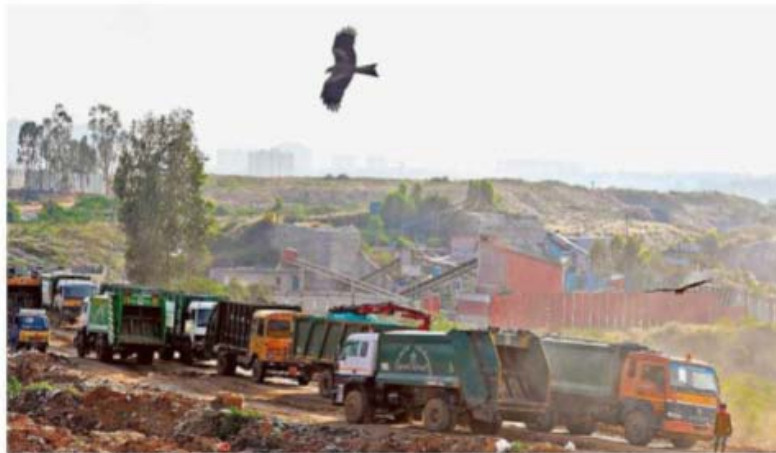
The garbage dumping yard at Mittaganahalli quarry pit. •SUDHAKARA JAIN
